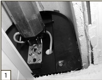
First, install the tubular motor in the roller shutter box in accordance with the tubular motor instructions.
