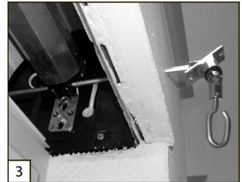
Push the articulated crank rod through the wall into the emergency motor drive.
