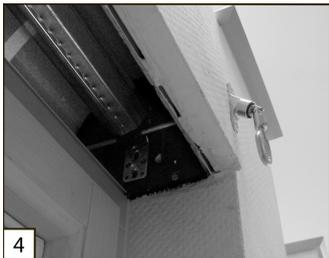
Fix the articulated plate to the masonry.
