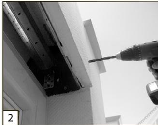
Then drill the hole to insert the articulated crank rod.
