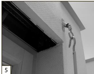
Attach the hand crank in the event of a power failure and open or close the roller shutter manually.
